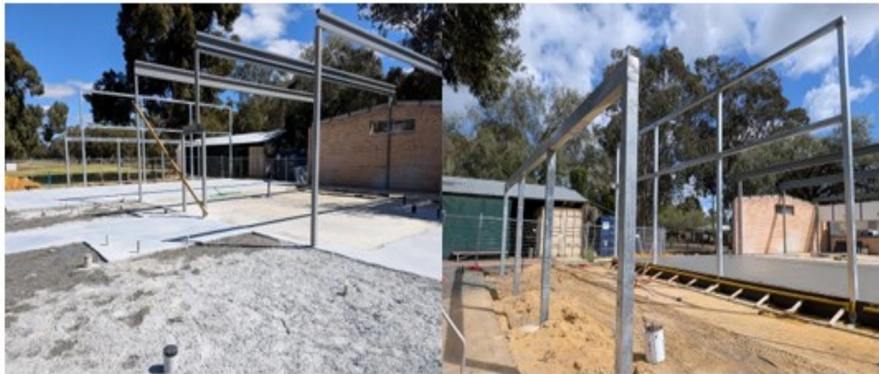
Structural steel columns and roof beams in place. Concrete slab poured.
