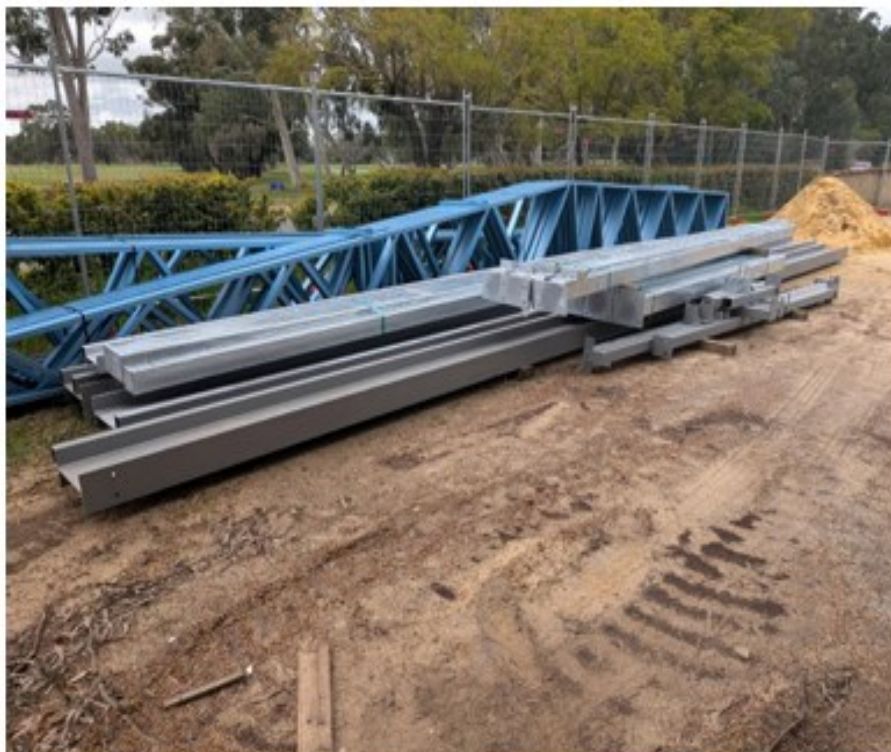
Steel roof trusses, structural columns and beams delivered to site.
